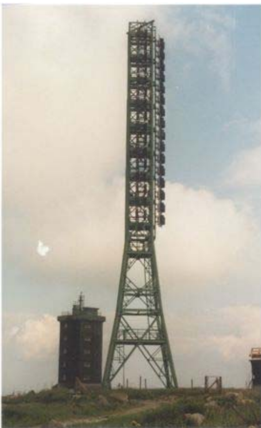
Illustration 21 High-gain reception antenna for the „Horizont“ system on the Brocken mountain, Harz highland
