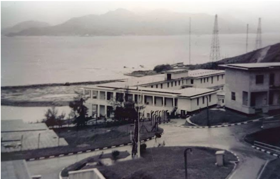
View of antennas at Little Sai Wan Hong Kong
