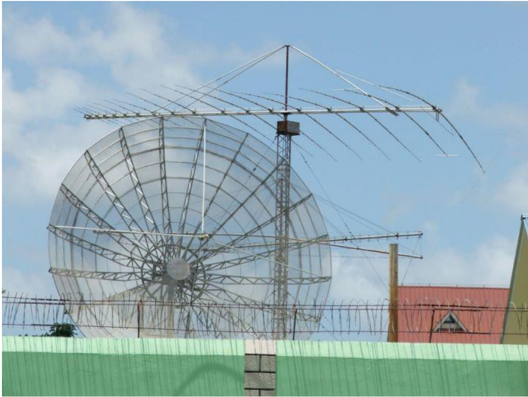
Two of the HF antennas [there are more along with V/UHF in the compound] and the satellite dish.
